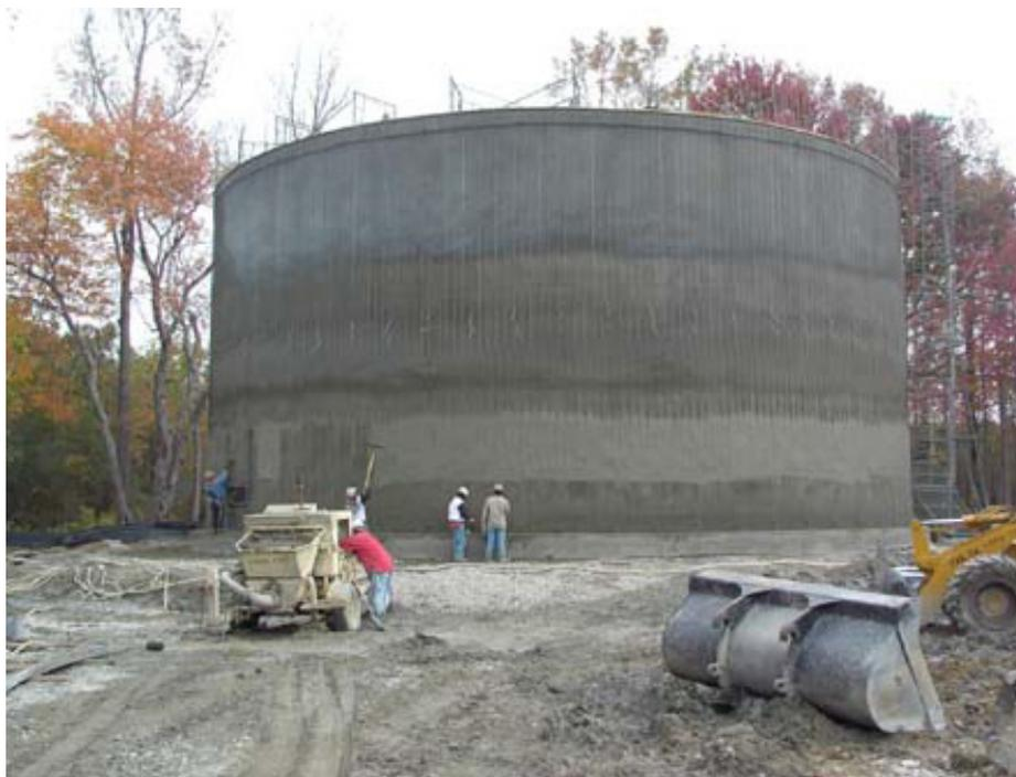
Fig 1. Sealit Multipurpose being applied to the outside of a large water tank.
